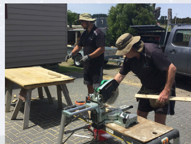
Left to right: 'Before' renovations. 'After' accessibility ramp, handrails and steps. 'The Handyman' Ross and Hedley Darling.
