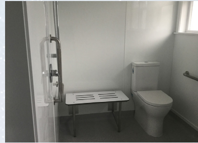
Left to right: Jan Rameka and Manu Vincent (Project Managers). Entrance steps and rails. Bathroom support features.
